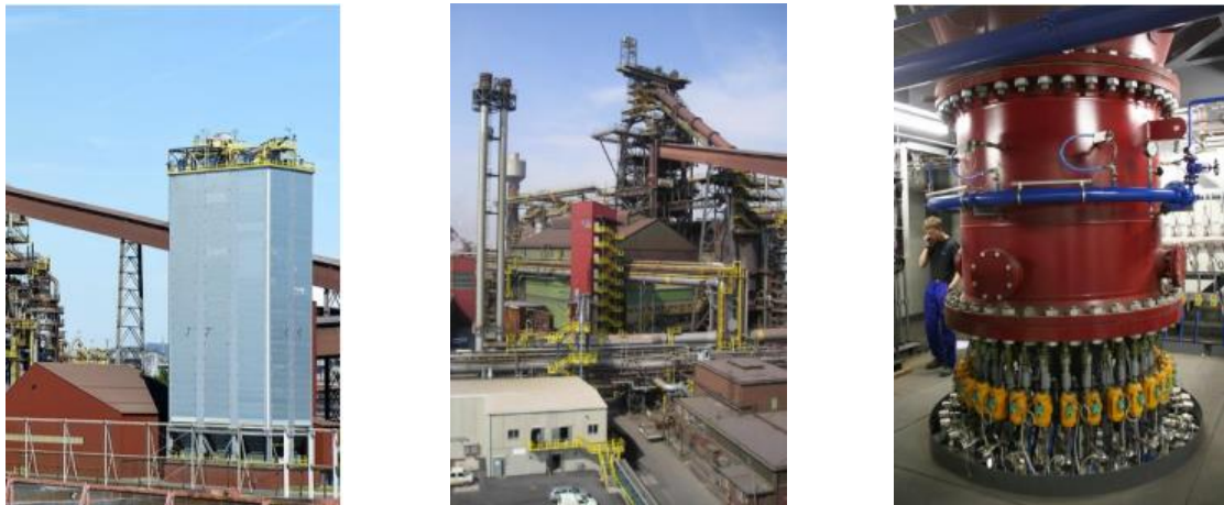
Figure 8: Plastic injection at BF A of voestalpine Stahl GmbH; Material handling and storage (left), process air compression and injection tower (middle) as well as pressure hopper and material distribution (right).
