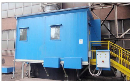
Sound-insulating housing for returning fan exhaust system to the sinter belt in the sinter plant
