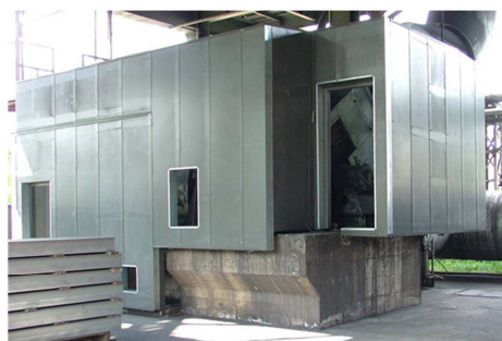
Sound absorbing and insulating enclosures on fans in dust collector in cokery
