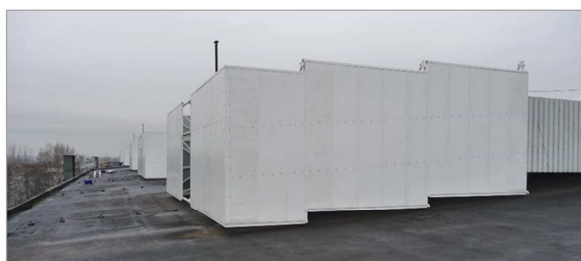
Acoustic screens for six skylights in cold rolling mill annealing plant
